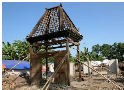
(a) Saka guru structure
